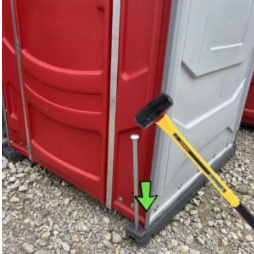
Figure 27: Photo showing staking of portable toilets to secure from tipping
